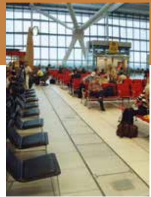
Above: Duct run with service access points within covers
